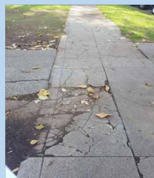
Immense amount of alligator cracking on the asphalt and sidewalk.
