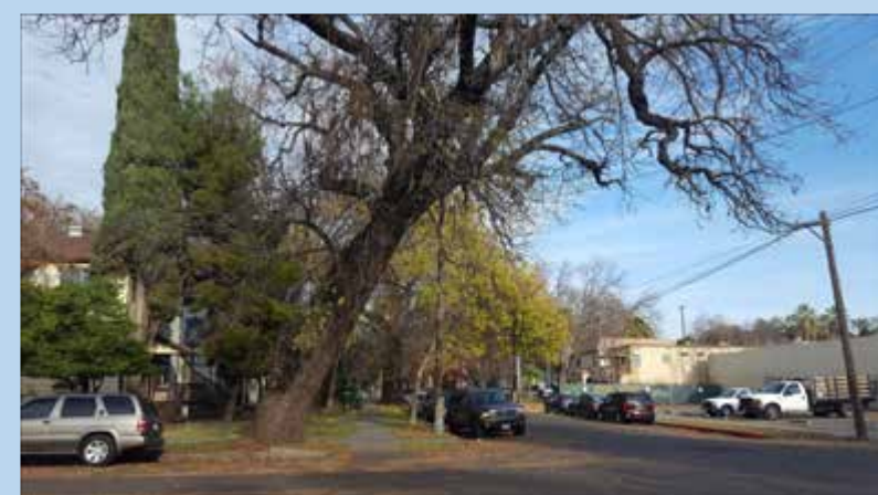
Large trees which may be safety threats due to large branches. Roots are also breaking through concrete and making pavement uneven.
