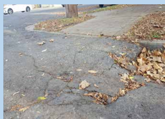
Immense amount of alligator cracking on the asphalt and sidewalk.
