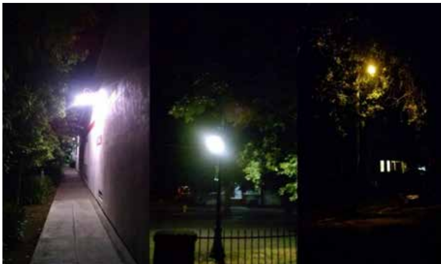
Figure 2. Effect of lamp Positioning; Illuminance of retail mounted light (left) Acorn style streetlight (center) and Cobra style streetlight (right)
