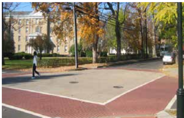
Figure 15. A raised intersection with a brick slope
