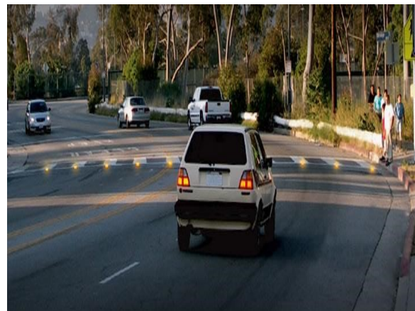
Figure 17. In-roadway warning lights during day time
