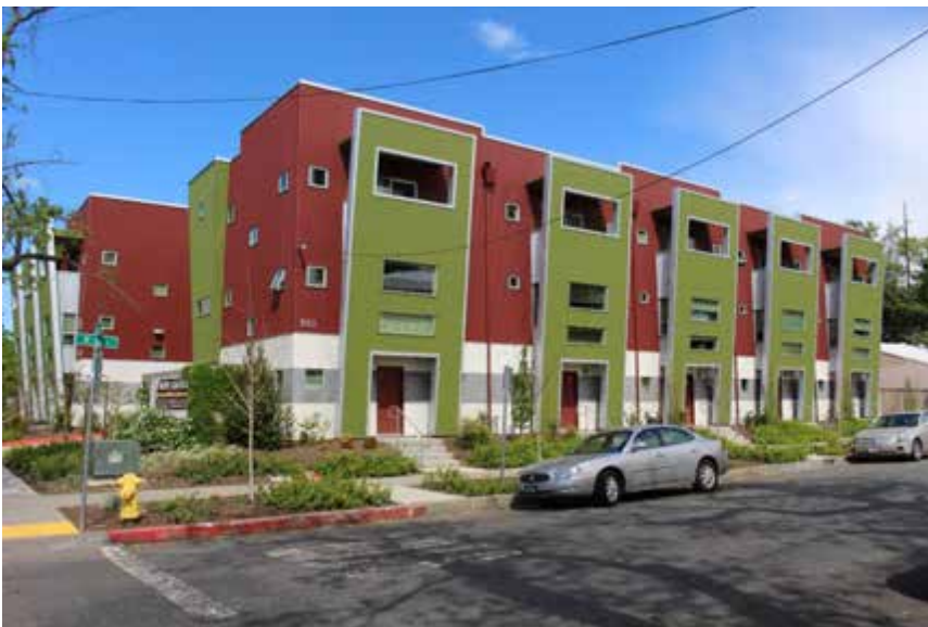
Portland Place Apartments, Orange St
